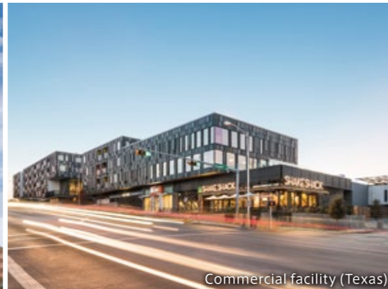
Commercial facility (Texas)
